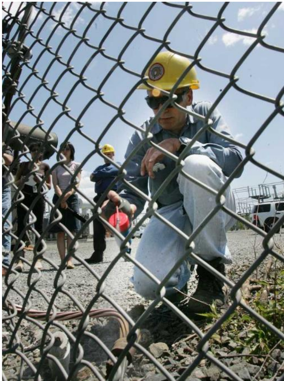
An NSP worker applies Datadot to copper wire at a substation in Halifax on Monday. (Daily News/Andre Forget)
